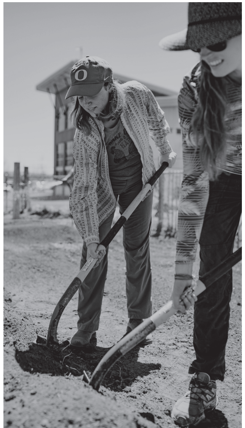
Hannah Ryckman, left, and Haley Morris shovel dirt to restructure plant beds at the Rec Center garden.
